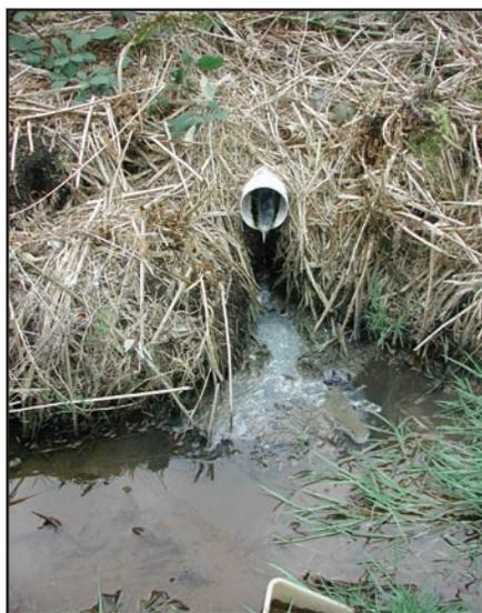
**Figure 2: Direct Discharge from a Straight Pipe**
